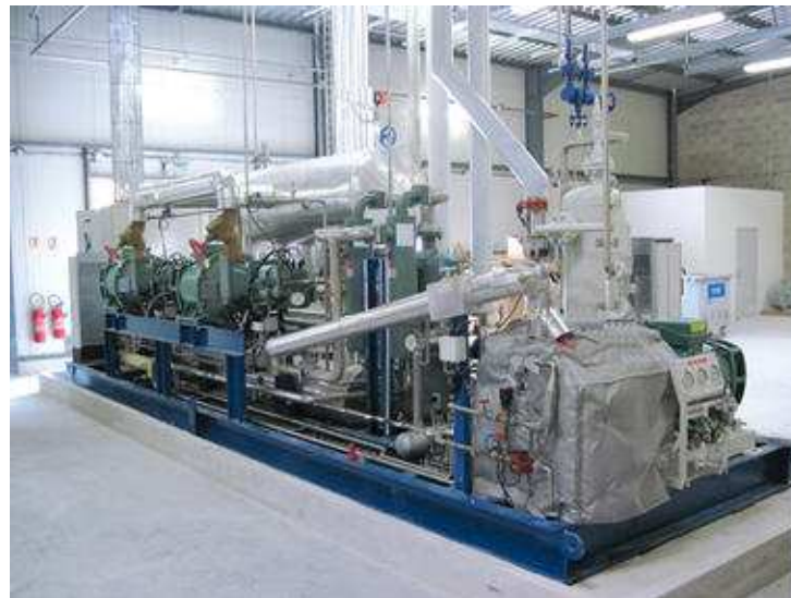
High Temperature Heat Pump developed for Dairy Industry.
